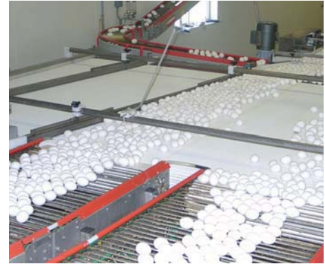
Installation of Curve Conveyor, Accumulator Table and Dirty Egg Return Conveyor
